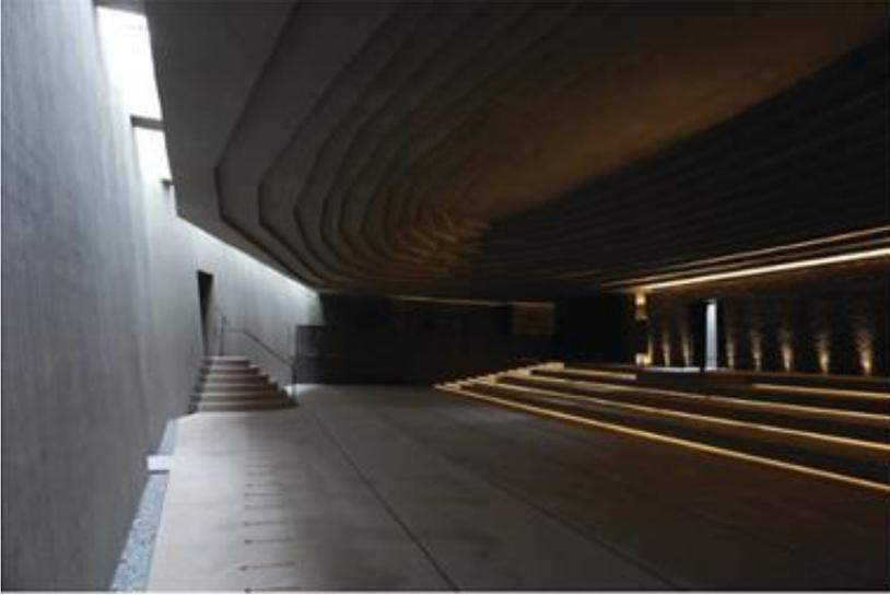
**Figure 4:** Disjunction between the qibla wall and the roof and slab of the prayer area (Gür, 2017)
